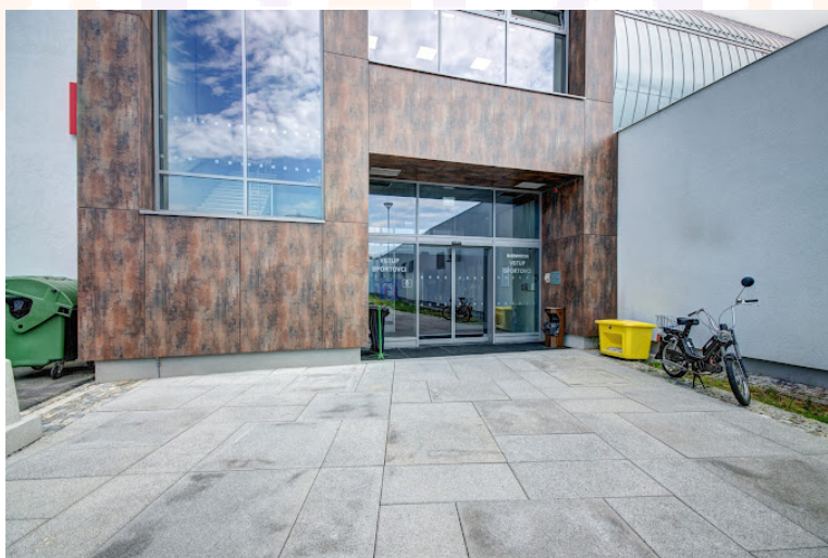
View of the back entrance
