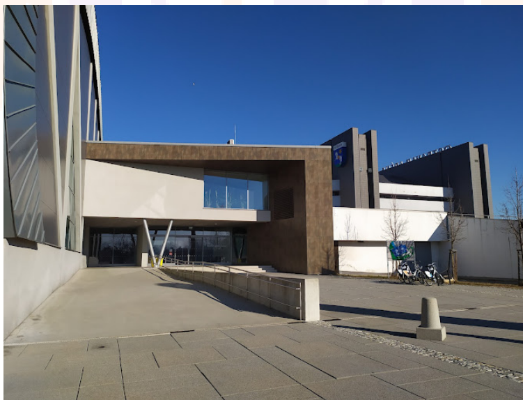
View of the main entrance
